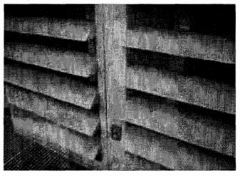
Fig. 5. It can be seen that the louvers are fixed in a horizontal position, painted white and are very dirty.
