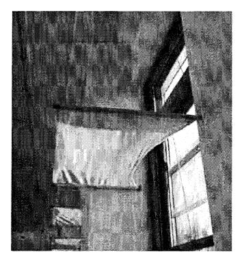
Fig. 15. A view of the shading device attached to the interior of the windows. It also serves as a daylight reflector/light shelf to bounce light up to the white painted concrete ceilings.
