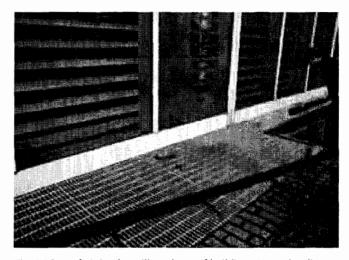
Fig. 4. View of air intake grille at base of building. Note clouding on center glazed unit.
