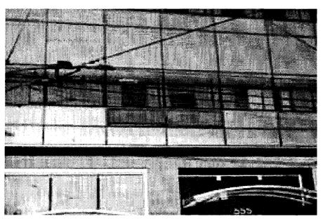
Fig. 8. Here we can see the differentiated glazing: clear versus fritted glass, and two of the operable windows in an open position.
