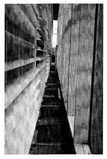
Fig. 6. A view inside the cavity showing its clear width to allow for maintenance; the plywood sheets that close off the grille at the base preventing air intake.
