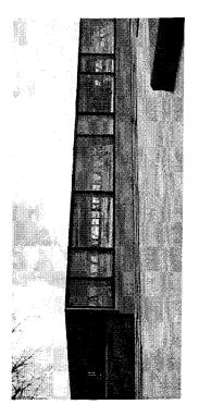
Fig. 16. A view of the side elevation of the attached double skin component. You can clearly see through the entire space and it is evident that the space in not compartmentalized. The structure that holds the curtain wall away from the existing concrete frame forms a lacelike network within the cavity.
